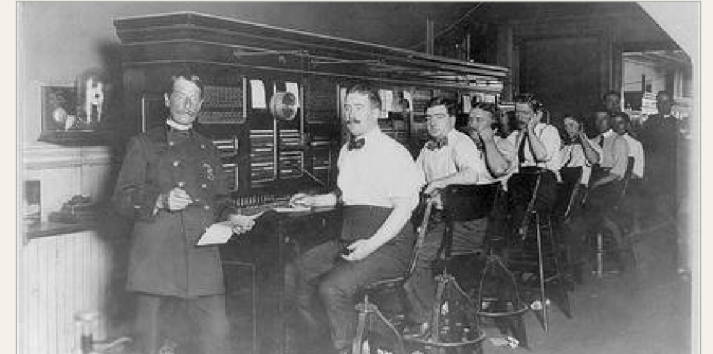
POLICE SWITCHBOARD, 1909 • LIBRARY OF CONGRESS
