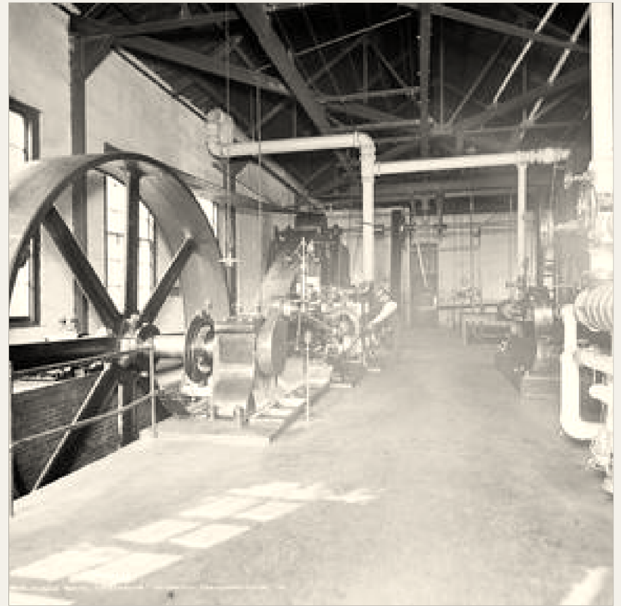
ENGINE ROOM, MERCHANTS' DESPATCH • LOC • LC- DIG-DET-4A11858
